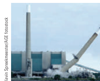
Figure 10.13 (Conceptual Example 10.5) A falling smokestack breaks at some point along its length.
